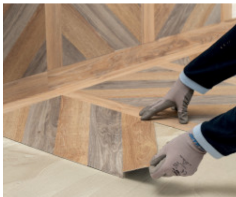
Installation of MODULAR LVT with Ultrabond Eco V4 Evolution
