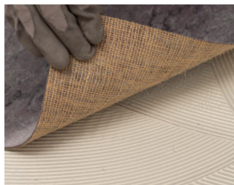
Installation of Linoleum with Ultrabond Eco V4 Evolution
