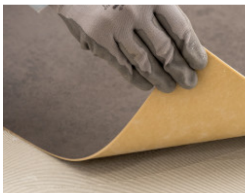
Installation of polyurethane-based flooring with Ultrabond Eco V4 Evolution
