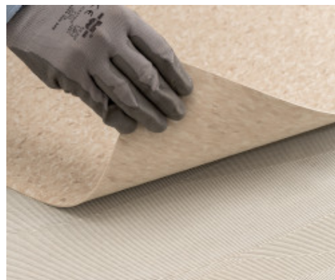
Installation of homogeneous PVC with Ultrabond Eco V4 Evolution
